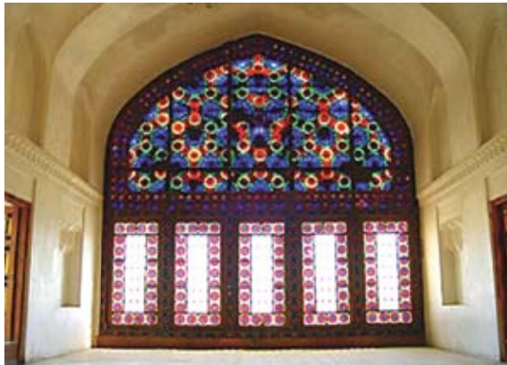
Figure 4. Hot-dry regions house windows
