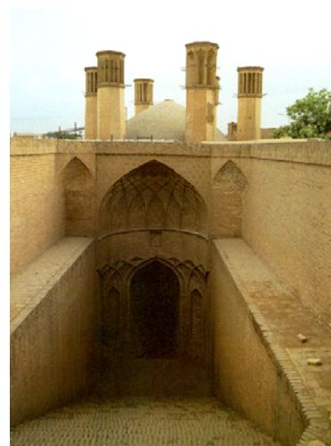
Figure 12. Six wind-catcher Abanbar in Yazd
