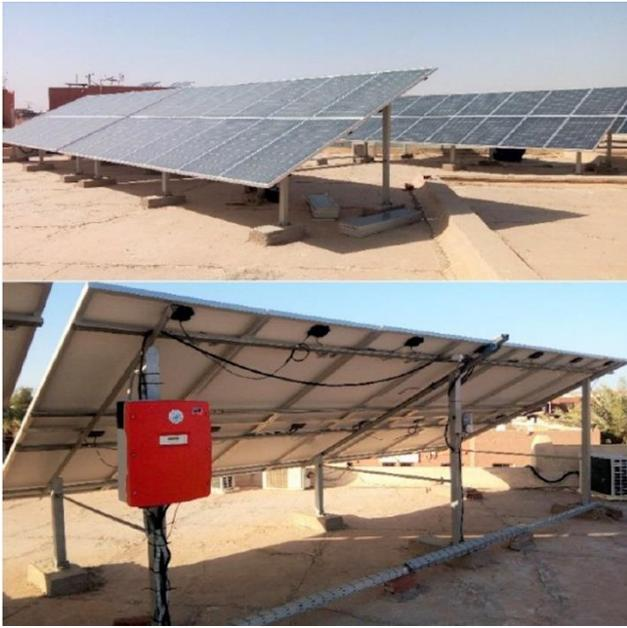
Figure 1. Scene of 10.5 kW PV module station [10]
