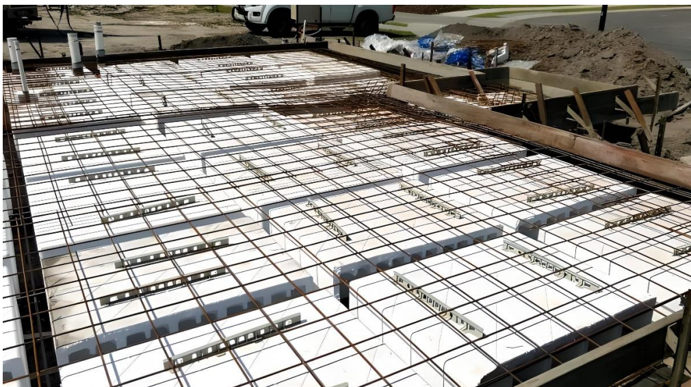
Figure 7. waffle-slab-construction-reinforcement [20]
