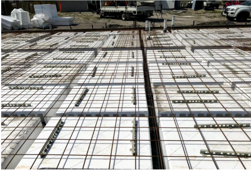
Figure 6. Meshing in waffle slab with solid sections [19]
