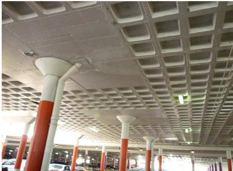
Figure 4. Analysis strips of the waffle slab with solid sections at columns [15]
