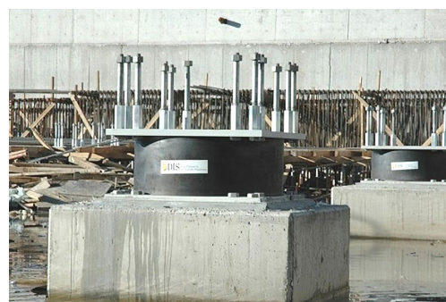
Figure 2. Elastomeric base isolation devices [4, 5]
